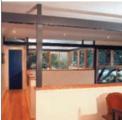
DuraGal Channel grade C450L0, 150 x 75 x 5.0 & 200 x 75 x 5.0 / 6.0 were used for the main floor and roof support members, with DuraGal SHS grade C450L0 65 x 65 x 5.0 for the stub columns.
