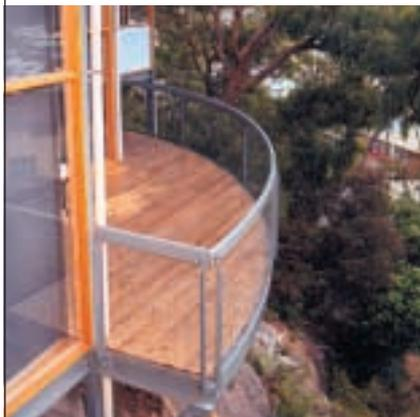
DuraGal Rail (a flat sided oval) is available in several sizes, the 120 x 48 x 2.0 Rail section was used for the upper handrail on the decks and entrance area.
