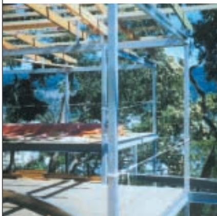
DuraGal Hollow Section grade C450L0, 90 x 90 x 2.5 SHS for both the full height and up to floor level columns (standard bottom footing plates and bracing sets from the DuraGal Flooring System were used).
