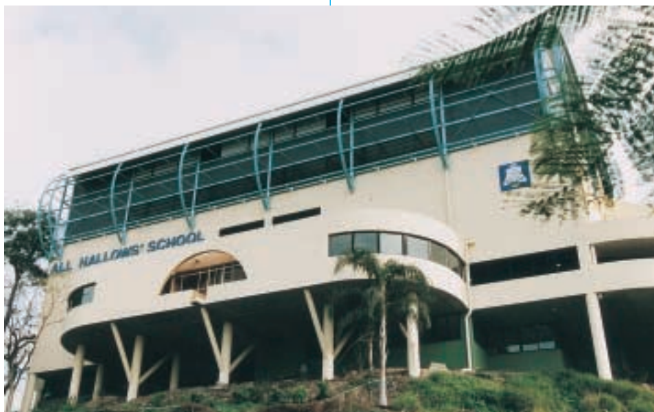
Steel-framed Mercy Hall sits lightly over concrete structure of Loretto Hall.
