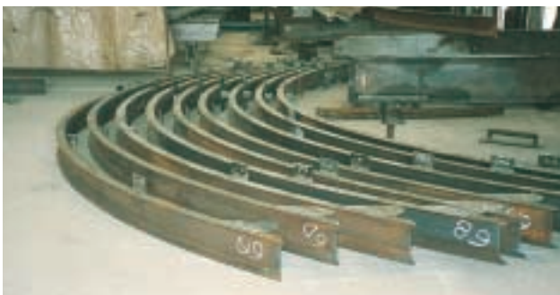
Left: 300PLUS 200x75PFC sunshade frames cold rolled to shape.
