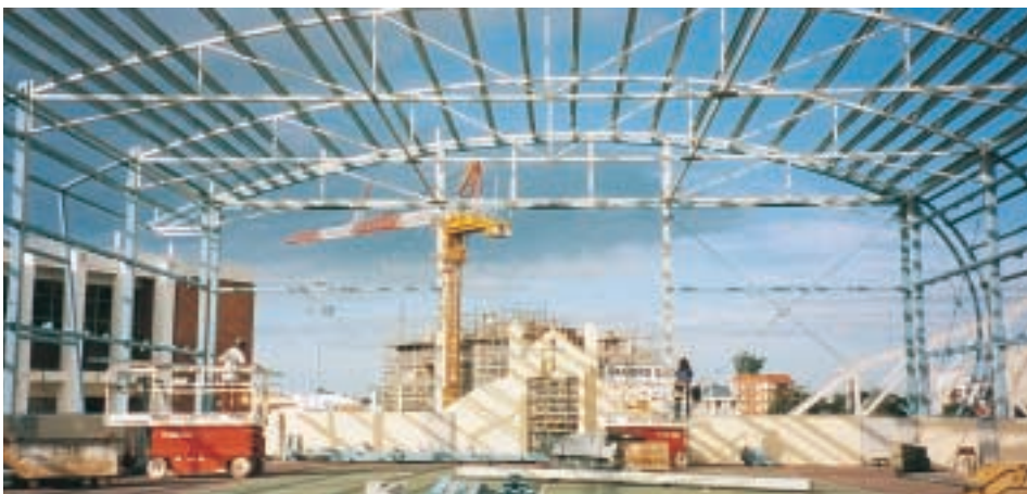
Below: Completed steel frame using scissor lift for connections.
