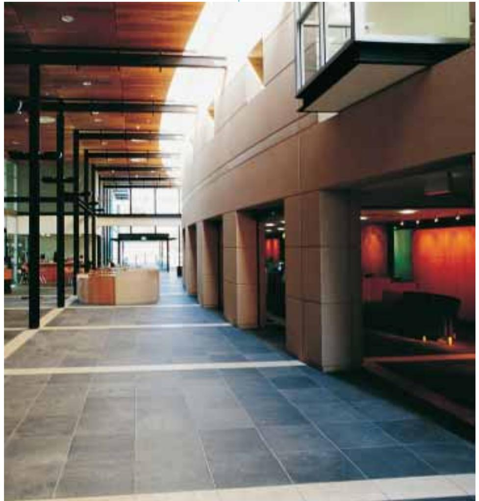
in a grid of 3.9 m giving a square format, both horizontally and vertically to the facade treatment. The exposed steel framing allows for different infill panels to be used, primarily aluminium framed glazing, interspaced with solid infill panels of compressed fibre cement sheets. They modularise the exterior appearance in addition to suiting the function of the internal spaces.
