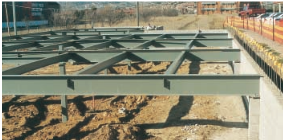
Underfloor steel framing, under construction.
