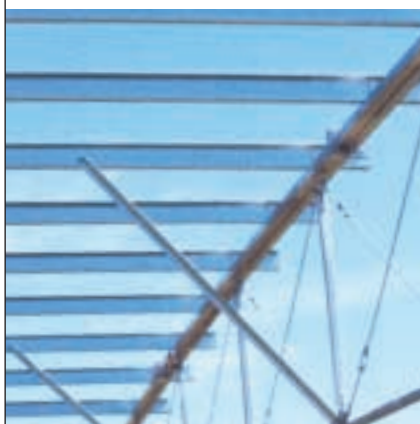
Fly Bracing: 65 x 65 CA DuraGal Angle C450L0.
