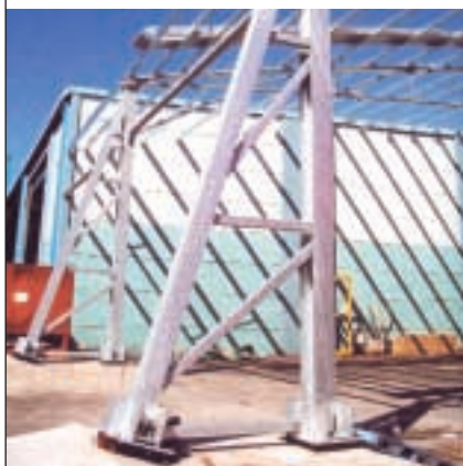
Columns: OneSteel 200UC & 250UC Universal Columns in a buttress open web form.
