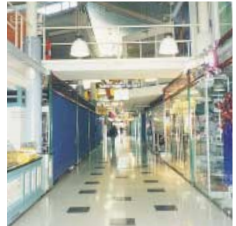
Original top floor showing narrow walkways and original plantroom above shop premises.
