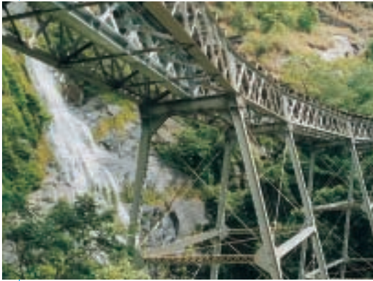
Above: Upgraded Stoney Creek bridge.
