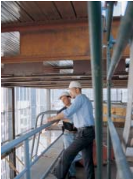
Steelwork on Level 16, showing web penetrations.
