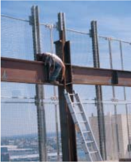
Erection of perimeter beams.
