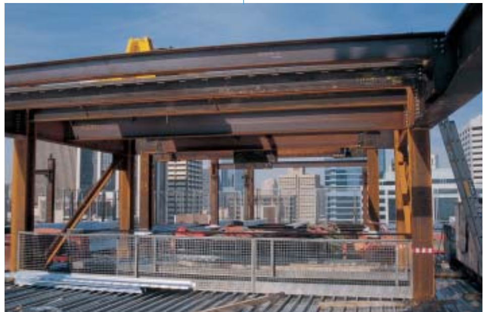
Diagonal bracing indicated core location.
