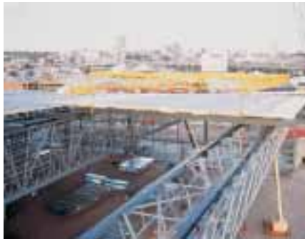
Panelised roof construction.
