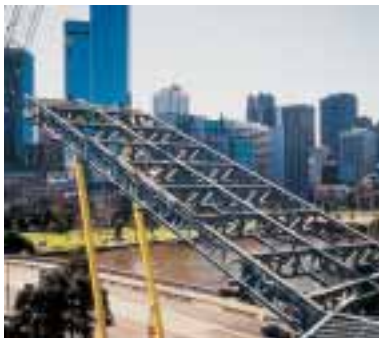
Top: Truss to column joint assembly.
