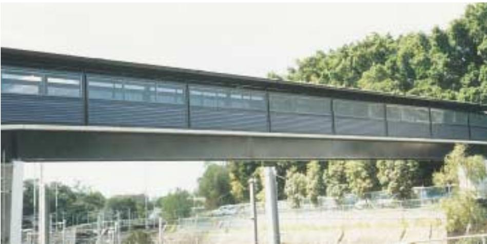
*OneSteel Welded Beams support the link between old and new at Brisbane Grammar School. A new steel pedestrian bridge spans 43m over the railway to the site of a new \$8.5M Indoor Sports Centre. The lightweight, long-spanning characteristics of OneSteel's Welded Beams were equal to the challenge of an inaccessible site.*
