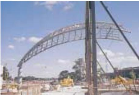
Top: Erection of the barrel vaults along the length of the railway station.
