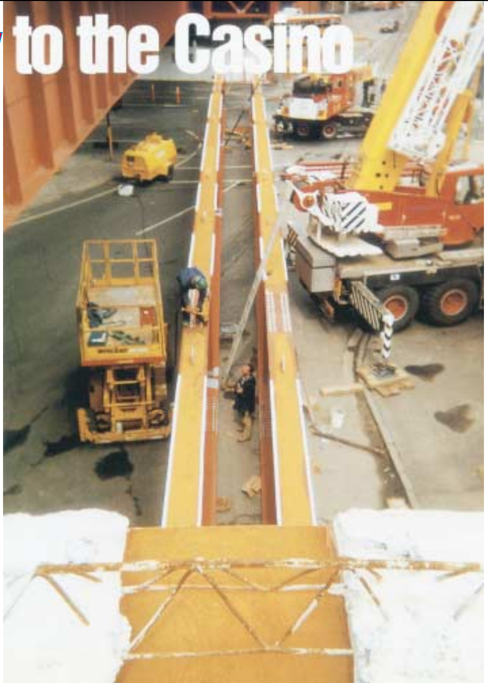
Girder segments being bolted together before lifting directly above.
