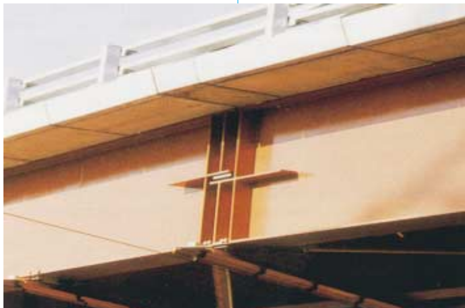
Left: Stepped joint with pot bearing for drop-in span.
