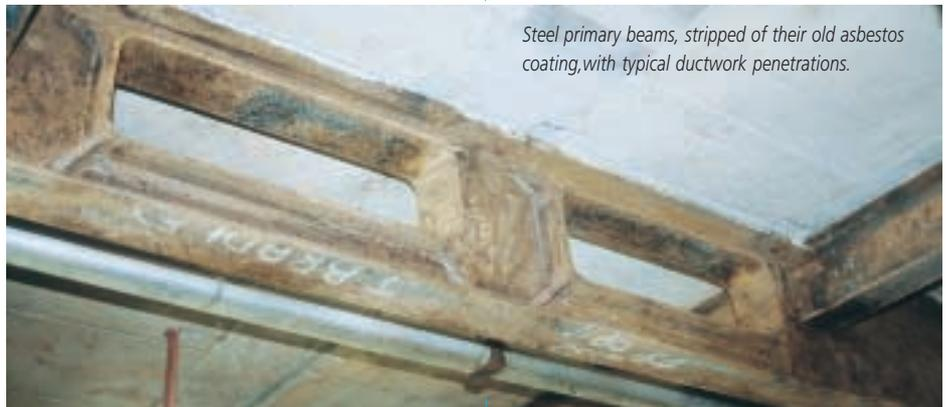
Steel primary beams, stripped of their old asbestos coating, with typical ductwork penetrations.
