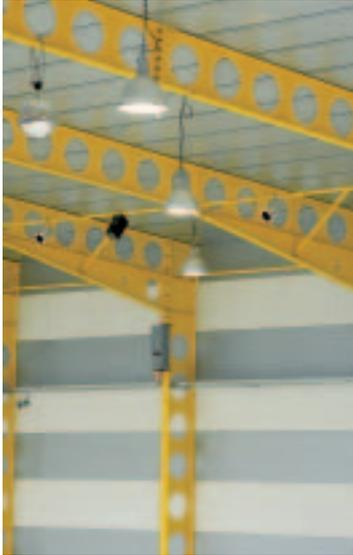
Peter Waugh of Low & Hooke Partners, the civil, structural, and hydraulic engineers on the project, said that: “The structural steel portal frame design was developed from the previous ice skating facility we built utilising Cellform castellated beams.”
