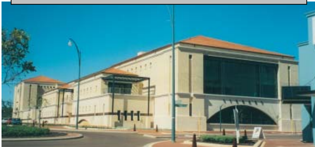
Stone exterior hides a heart of steel at Joondalup Civic Centre.
