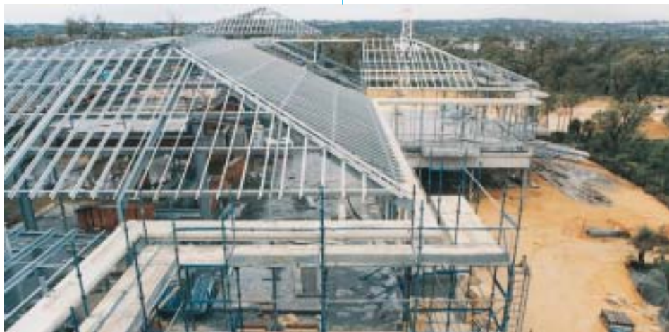
Steel roof framing on Council Chamber.
