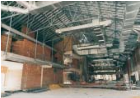
Top: Steelwork to double storey Council Chamber above concrete podium.
