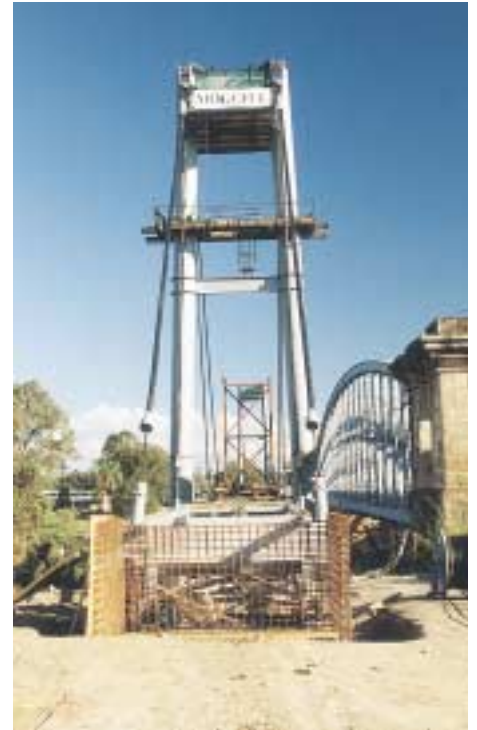
Tower and deck during construction.
