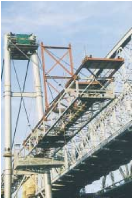
Tower and deck with lifting frame.
