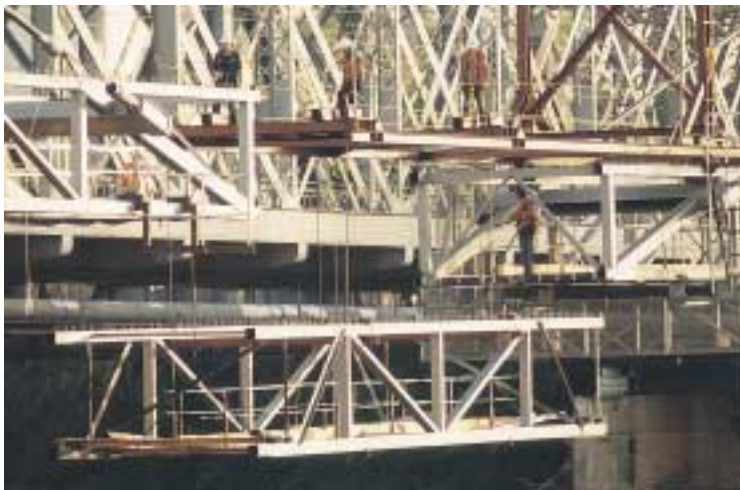
Final truss segment being hoisted into place.
