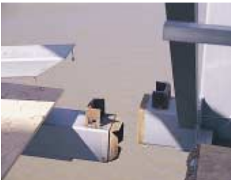
Truss segments about to be spliced.
