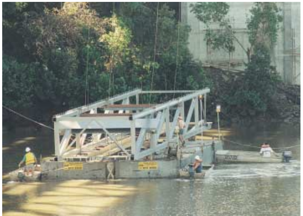
Truss segment on barge prior to lifting.
