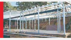
Wind pressure produces horizontal loads on the DuraGal Flooring System. For free standing floors these loads are transferred to the footings through the use of sub-floor bracing.
