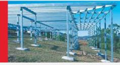
Difficult or sloping site construction can be easily handled by the DuraGal Flooring System. Developed by OneSteel, the DuraGal Flooring System is a steel flooring system utilising the higher strength and lighter weight advantages of DuraGal Hollow sections. The DuraGal Flooring System is suitable for a wide range of single storey residential homes, decks and commercial floors.
