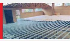
Whether the DuraGal Flooring System is used in brick veneer or free standing construction, assembly is straight forward and uncomplicated. The following is a typical step by step procedure.
