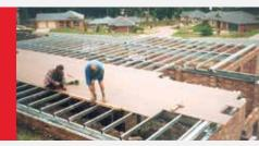
For brick veneer construction, there are many ways of fixing the DuraGal Flooring System to the brick work. The method used depends on the wind category and building preferences.
