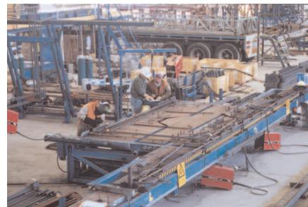
Above left: All reo was delivered to site in cages up to three times a day. Left: Materials were colour-coded to ease identification and special jigs were used to weld up the frames (right), and assist the steelfixers (below).
