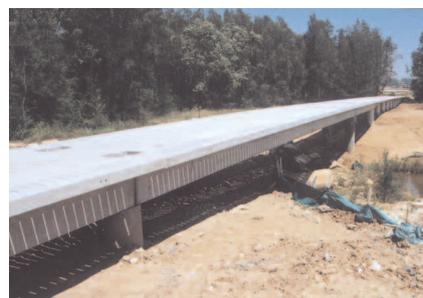
Left: The majority of bridges on the project used conventional precast bridge decks, as does the M7 cycleway.
