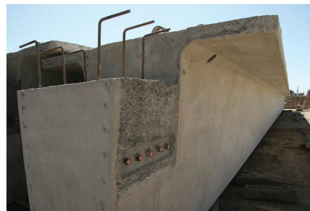
OneSteel Reinforcing provided privately owned Brisbane based company ENCO Precast with 500PLUS® REBAR and ONEMESH® Special Mesh solutions that reduced labour and added to construction efficiency of the reinforced concrete girders for the new 2.7 kilometre Houghton Highway Bridge duplication.
